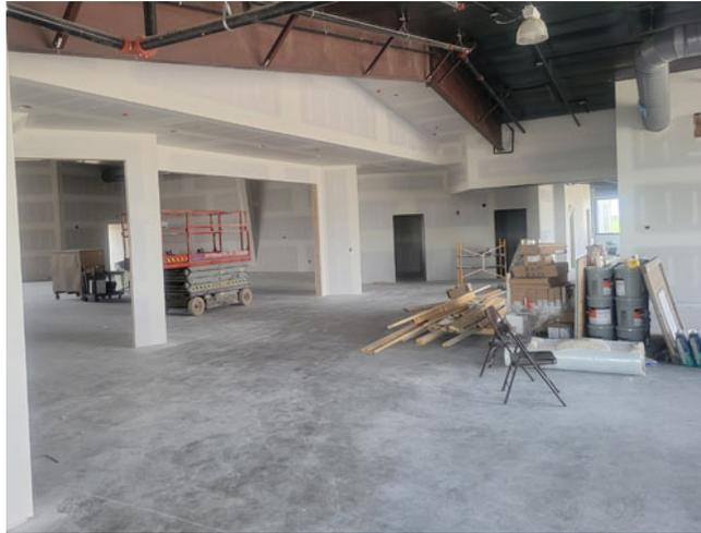
The administration wing is similar to the sanctuary. The insulation is in, the drywall is up, and next steps are texture, paint, ductwork and ceilings. Then floors, doors, and trim will have to follow as well.
